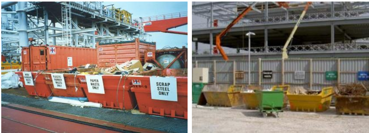
Figure 38. Examples of waste segregation at construction sites 68
